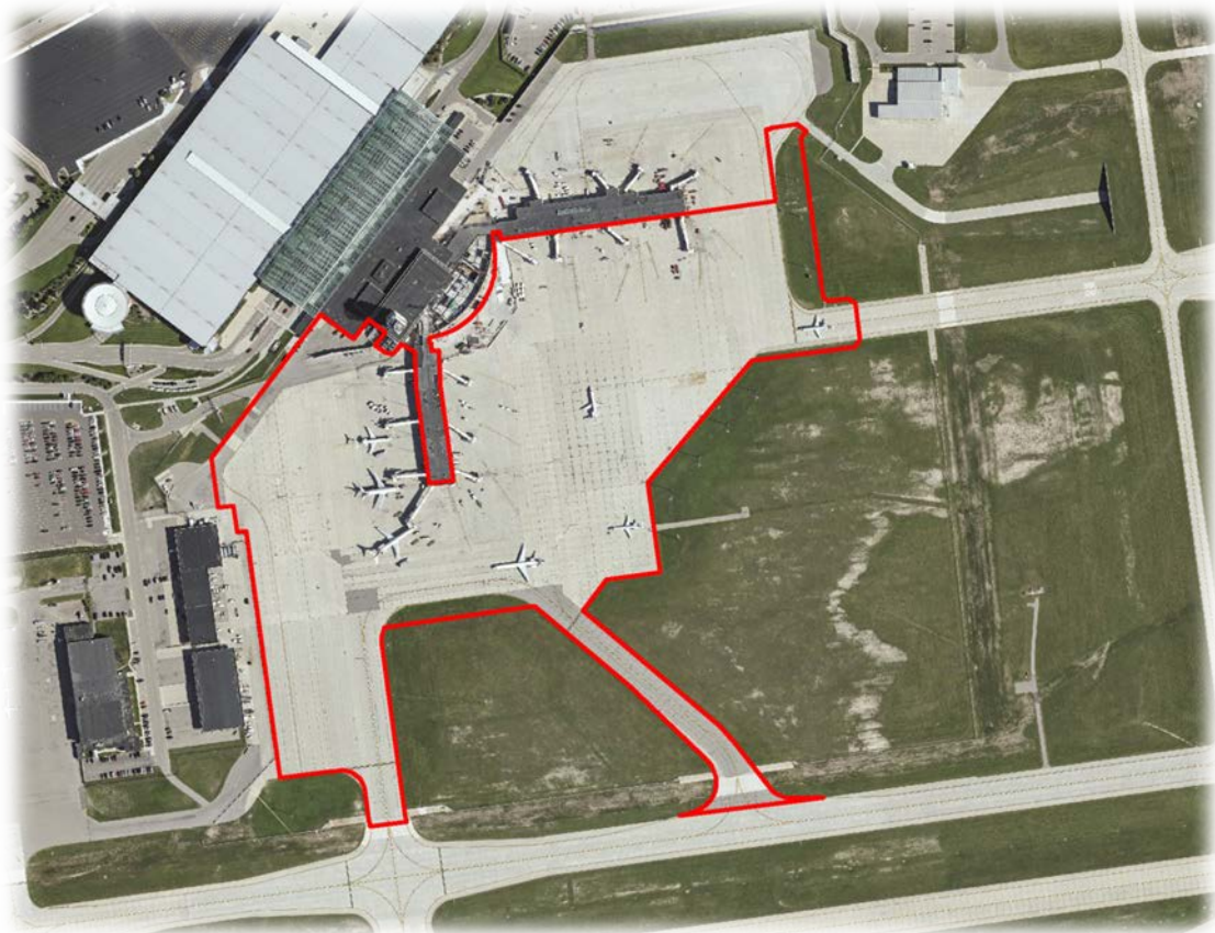
(Above): An aerial view of the Gerald R. Ford International Airport's apron reconstruction project and areas of construction shown in red.
