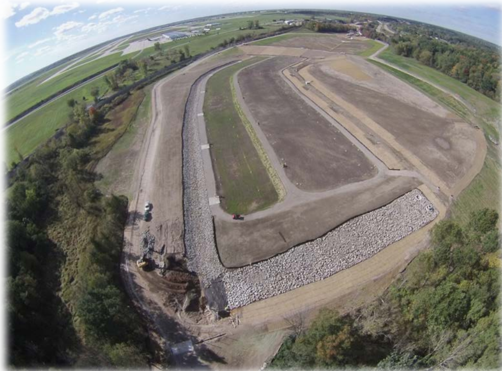
An aerial photo of the Gerald R. Ford International Airport Stormwater/Glycol Treatment System
