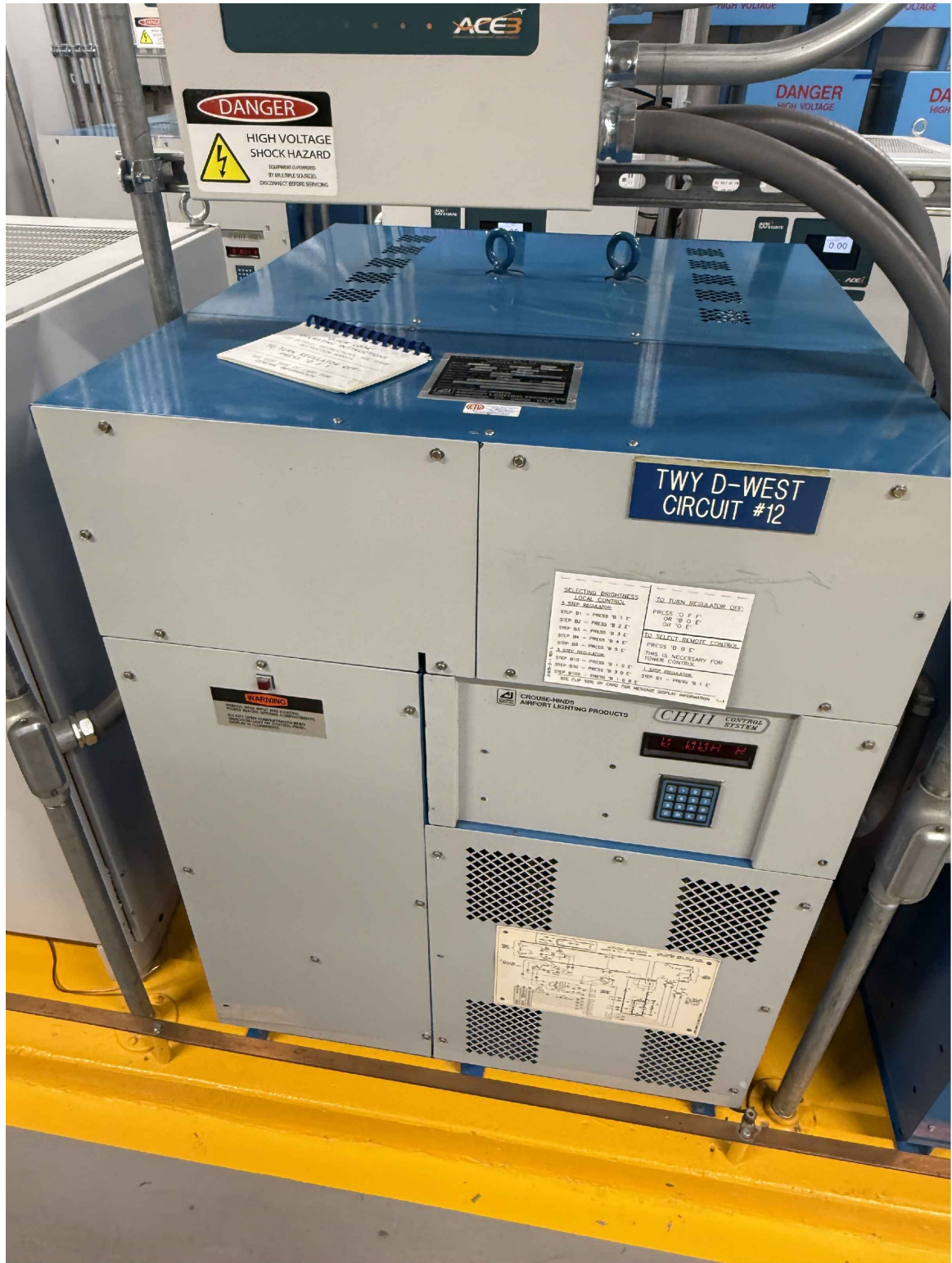
2 E302 EXISTING TWY D-WEST REGULATOR SCALE: N.T.S
